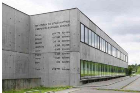
Lara Almarcegui, Matériaux de construction, Campus de Beau-lieu, Rennes , 2014, paint, 508 x 395 cm. Commission realized as part of the New Patrons Program of the Fondation de France. Production and mediation: 40mcube and Eternal Network. Photo: André Morin.
